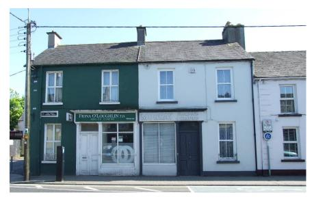
Fig. 94: Typical slate roof detail without overhang at eaves and verge on structures on Leinster Street
